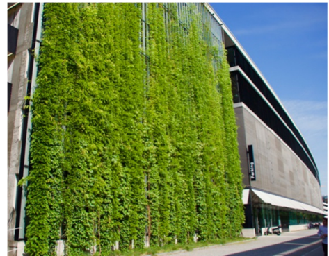
Figure 1 A example of a green façade on a commercial building (cable-supported green façade, Switzerland)
